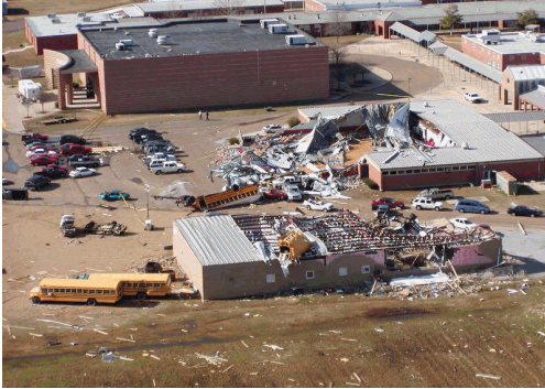
Tornado Damage - School Gym & Classroom Bldg.
