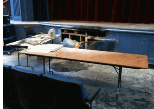
Fire Damage - School Auditorium
